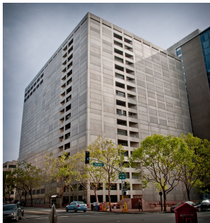
AT&T Switching Center, 611 Folsom Street by Remo Corso @t@ from wikimapia.org
